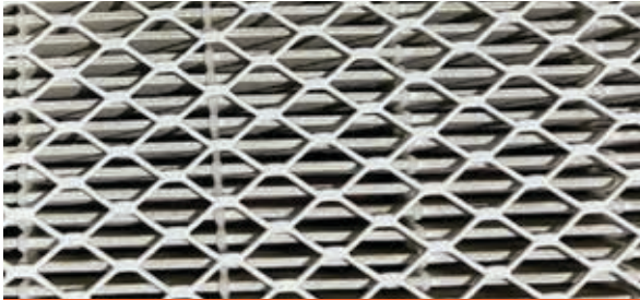
Figure A: Post FFU removal, ULPA filter upstream
