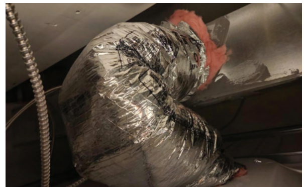
Connections with flex duct were completely kinked
