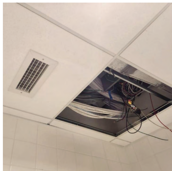
Exposed wiring visible where ceiling tiles were not installed
