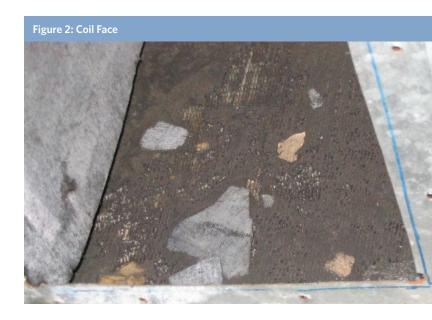
The RCx project was temporarily halted while the owner marshalled a quick fix team to clean all of the reheat coils, clean all crossflows, and install wire mesh at the workbench opens to prohibit papers from being sucked into the system.
