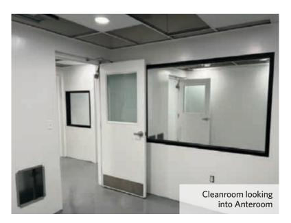
anteroom and four separate cleanrooms. It is being served by a Trane air handling unit with hot and chilled water coils. There is a total of 12 Fan Filter Units, 2 that are ducted and 10 that are not. They will be controlled by a SAMlink Control System which provides global, individual, and per zone fan speed adjustment and monitoring. It will also include a Gateway that will
