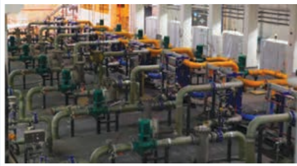
Figure 7: Inside the data center cooling plant rows of pumps flank their associated heat exchanger
