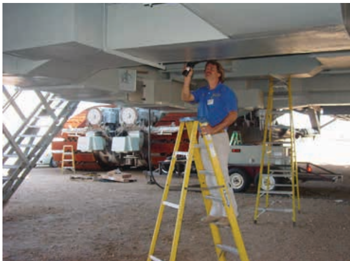
NASA Crawler Upgrade project: Curtis Smart of Thermal Systems Balancing Inc setting outside air at louver serving the operator "driver" control room.
