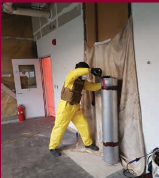
Worker with PPE and ballistic gear working on a decontaminated duct (flushed 24 hours).
