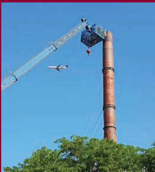
Stack that needed to be flushed accessed thru a mechanical lift.
