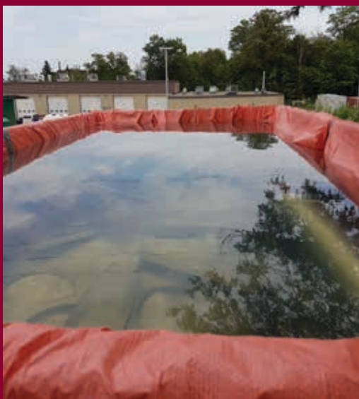
Lined tank filled with mechanical ductwork, soaking in water for perchloric deposits.
