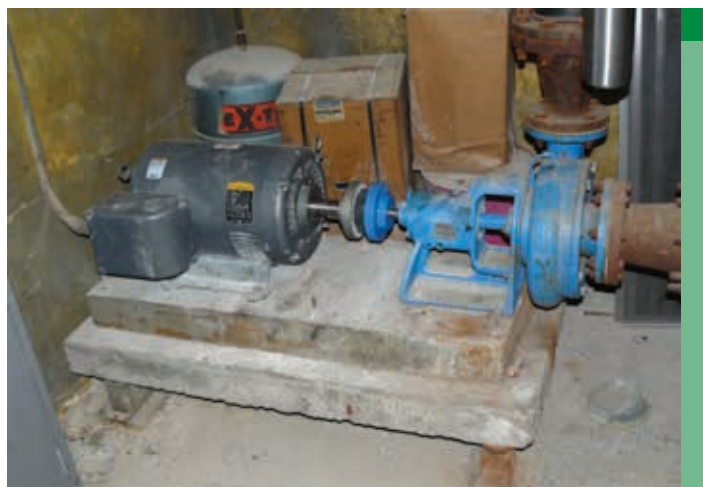
Figure 1. Re-Circulation Pump and Drive Motor Assembly
