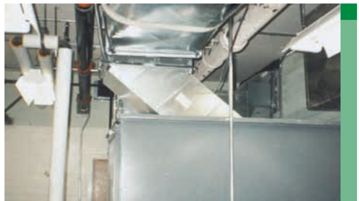
Figure 6. Offset installed in the turbulent area of a fan discharge
